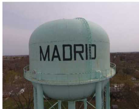
This 500,000-gallon legged tank was one of two tanks rehabilitated in Madrid, Iowa. The rehabilitation of this tank included several AWWA and
