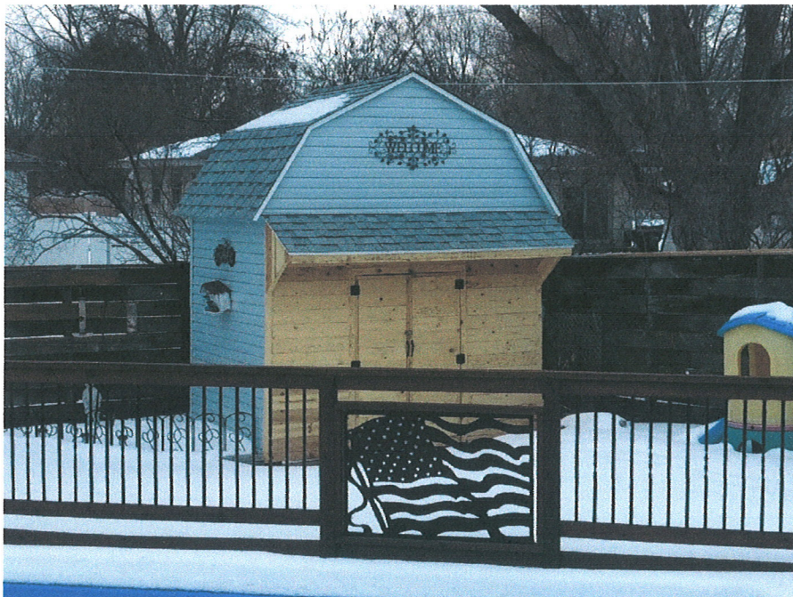
EXISTING PUMP SHED (siding and shingles match house)
