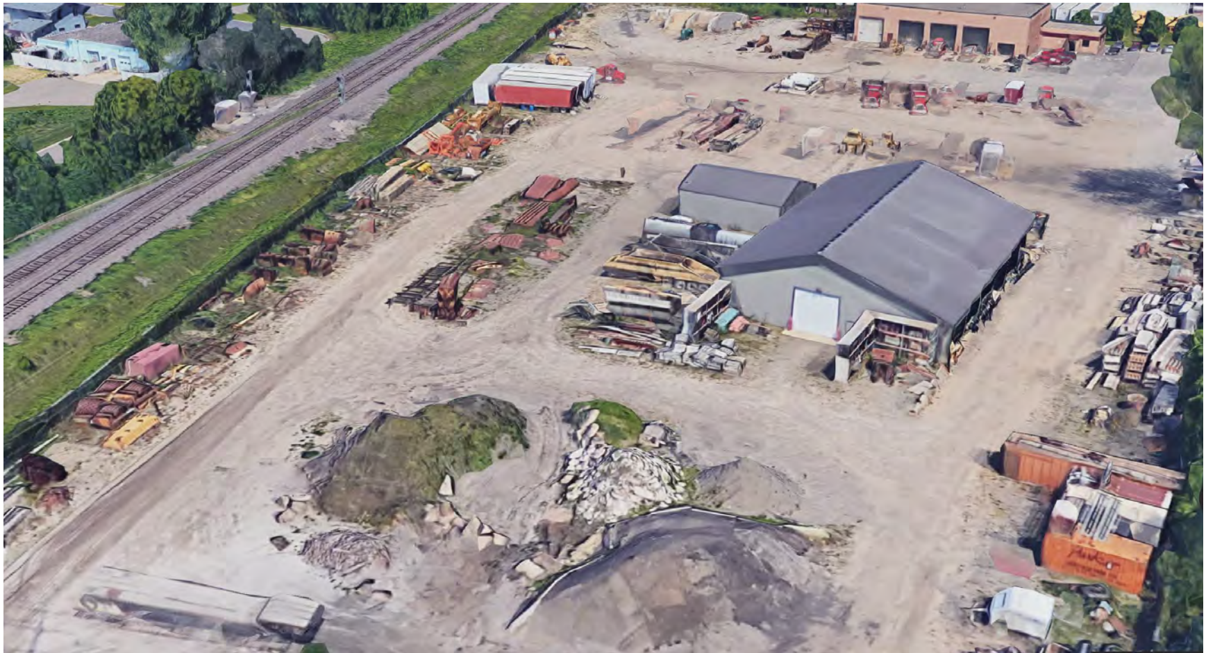
PARK CONSTRUCTION CURRENT STORAGE YARD - 30 81ST AVE NE
