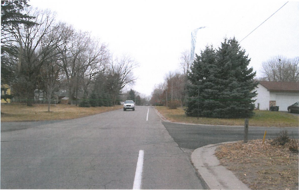
91 st looking west at Tyler
