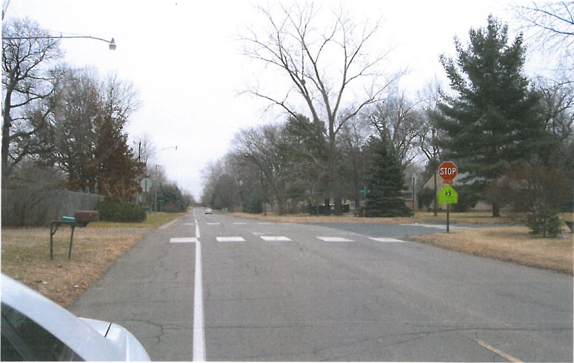
91 st at Jackson St looking east
