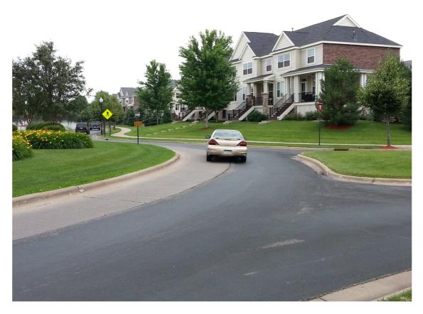
Newer roundabout designs feature a surmountable curb which separates the inner apron from the drive lane. This creates an uncomfortable jolt or bump to a passenger vehicle trying to cut the inside corner, forcing them to take the intended drive lane and travel slower around the roundabout yet still allows large trucks and semi-trailers to easily navigate the roundabout using the apron for the trailer wheels.
