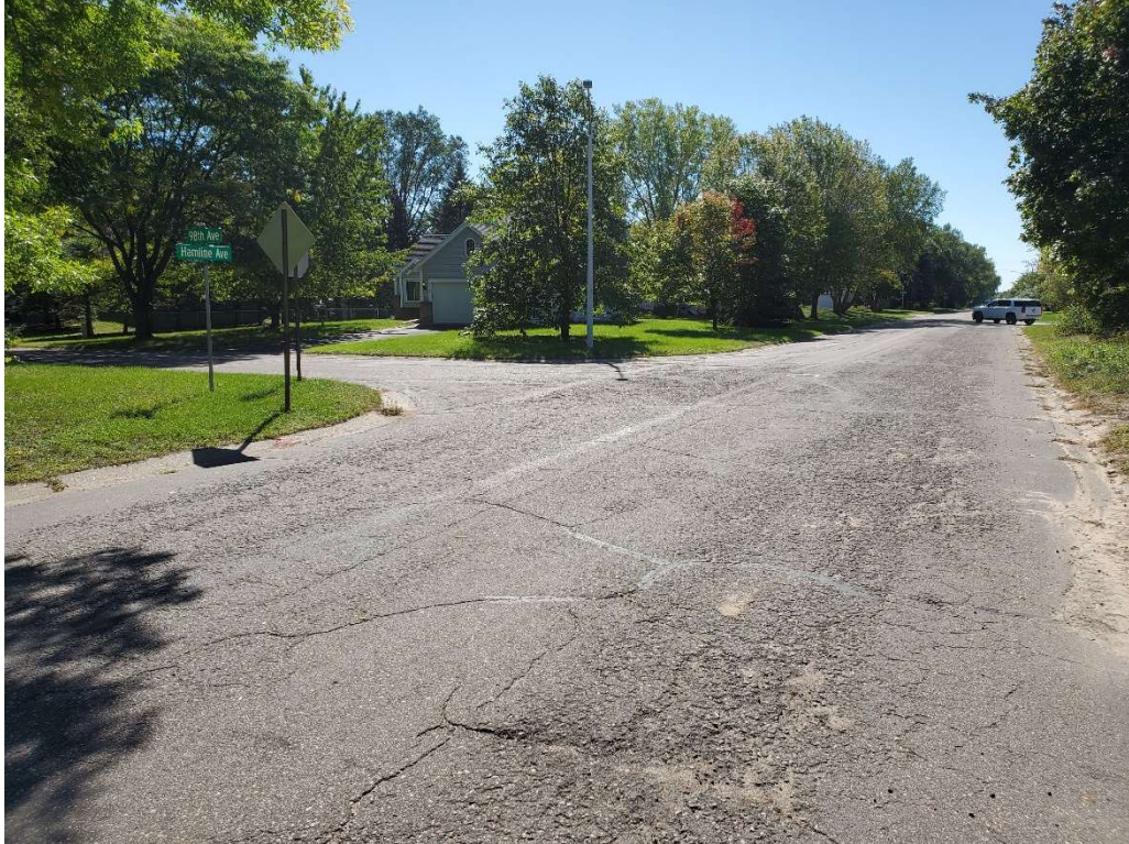
Existing Conditions at Hamline Avenue and 98 th Avenue
