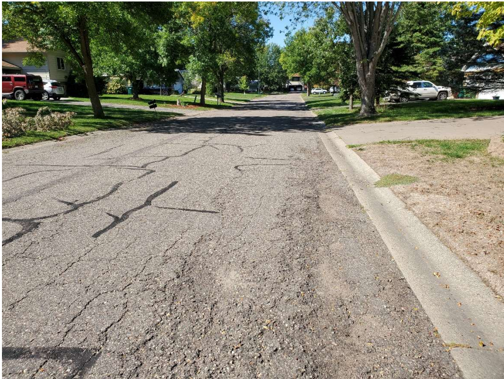
Existing Conditions on Yalta Street
