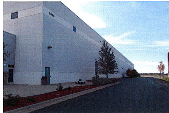
6 PHOTO OF EXISTING WEST SIDE-ADDITION TO MATCH EXISTING SCALE
