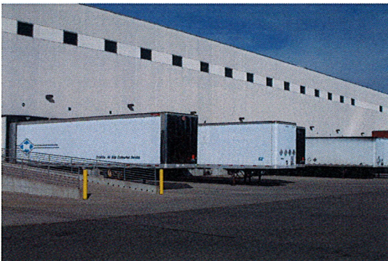
5 PHOTO OF EXISTING EAST SIDE-ADDITION TO MATCH EXISTING SCALE
